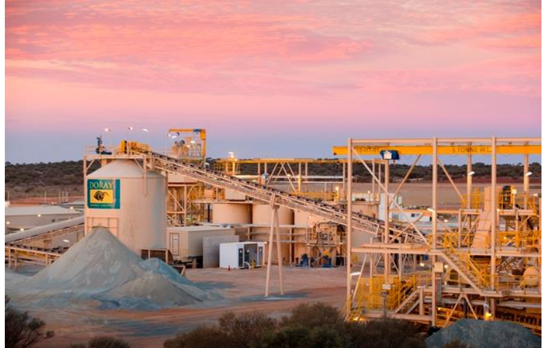
GR Engineering's Andy Well Processing Plant Project Image Source: www.gres.com.au
